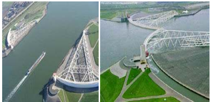
Rotterdam Flood Gates protect a channel 1181 ft wide and 75 ft deep
